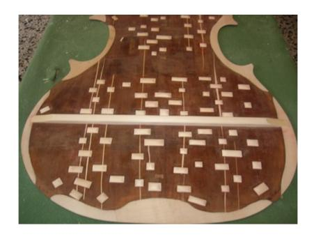
The glueing surface of the soundpost bar shows signs of at least two previous bars.
