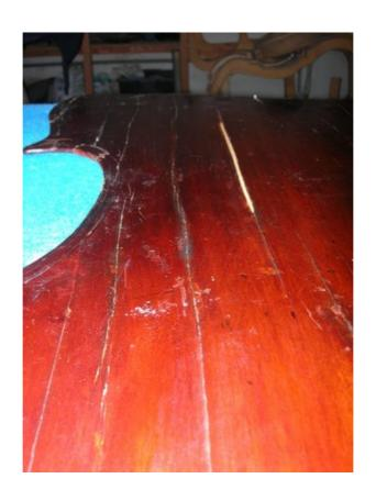
I remove the temporary cleats and clean the crack.
