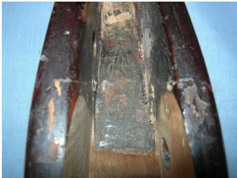
I thought completely remove the remainings of the old graft from the back of the peg box.
