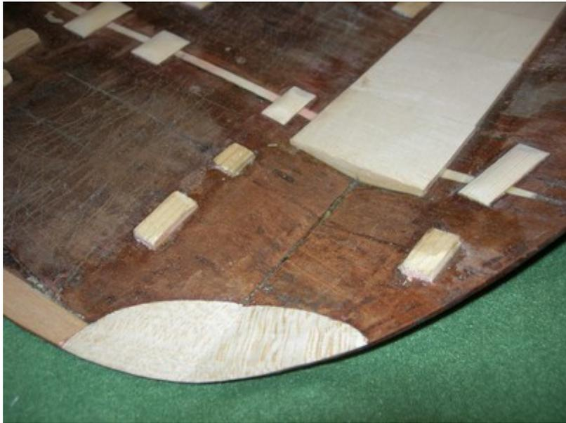
In the lower treble part there is a last crack, between the lower edge and lower corner, properly repaired with a shim, well glued.
