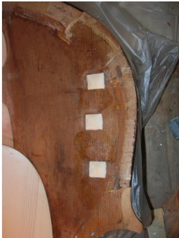
I place a temporary cleat to block the two cracks, properly closed, next to the center doubling, in an area that has been thinned to 2,5 millimetres, that will need a doubling.
