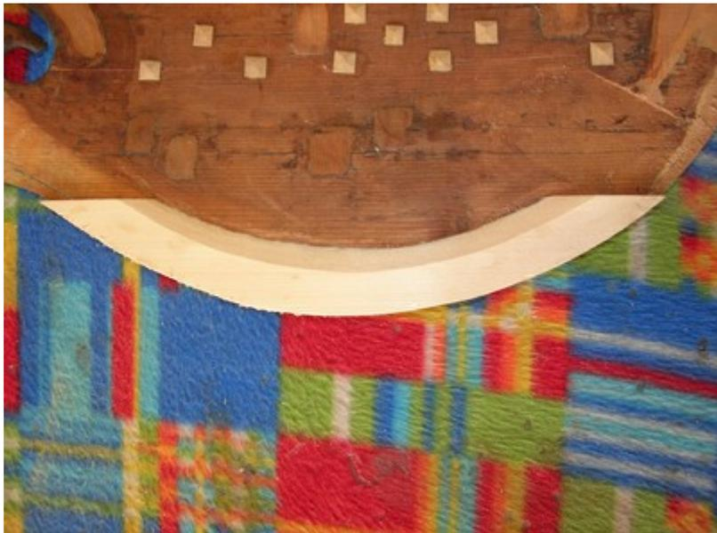
I remove the cleats, clean and repair the first two cracks, and put new cleats.
